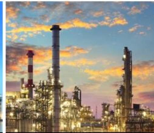
Combined Heat & Power
